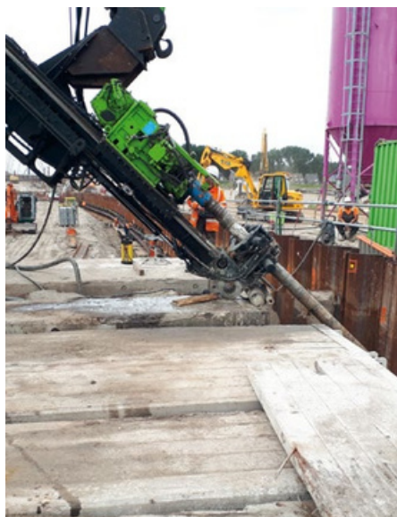
VD150 drilling 177.8 mm casings for strand anchors, 60 m long
