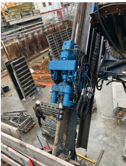
VD150: retraction of hollow bars, 60 m long
