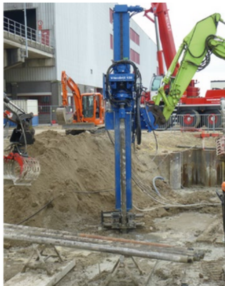
VD100 drilling in sand and gravel, 65 m deep, hole diameter 190 mm, flushing with water
