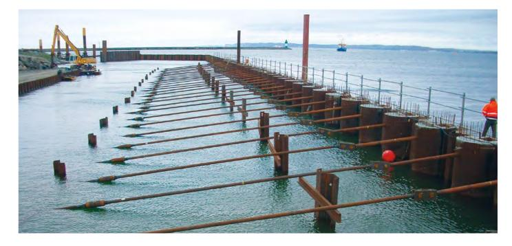
The solution for sheet pile walls: round steel tie rods. An anchorage employing round steel tie rods is an economical solution for securing a sheet pile wall, which can be adapted to suit the situation. The forces acting on the wall are transferred via the waling to the round steel tie rods and then to the anchor plates or walls. The selection and design of the anchoring structure is done in accordance with static and structural requirements.
